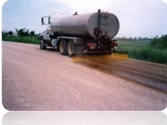
The photo above shows the application of dust control materials on a gravel road.
