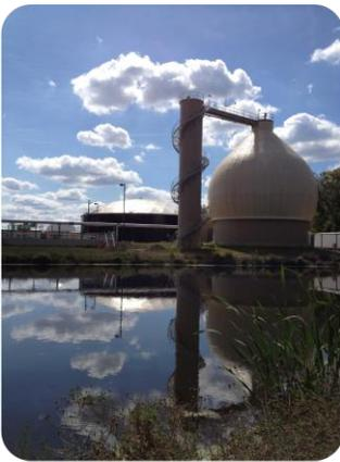
One of the innovative design features of the Grandville Water Plant is Michigan’s first Egg-Shaped Anaerobic Digester, with gas cleaning, cogeneration, and hot water recovery systems.
