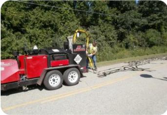
The above picture shows Calvin Top from the Hudsonville garage placing crack filling material.
