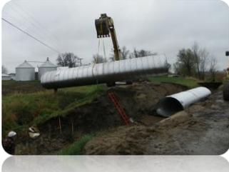
Shown above is the contractor My-Con installing a new aluminized culvert on 96<sup>th</sup> Avenue.
