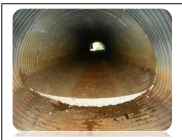
Shown above is the application of the experimental waterproof spray filler within a corrugated metal pipe culvert joint.
