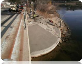
The above photo shows the concrete slope protection repair on the Green Street Bridge over Sterns Bayou in Robinson Township.
