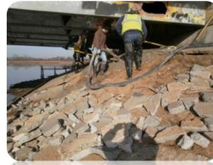
The existing concrete slope paving of the bridge was damaged by some vandalism.
