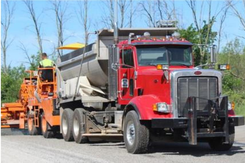
Seal Coat Surfacing (also known as a Chip Seal) is a perfect tool for pavement preventive maintenance.
